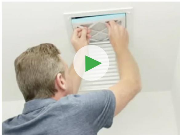
**The Lesson:** When installing air filters in HVAC systems in the dental office setting, choose the highest possible MERV level that the HVAC equipment can accommodate. If the HVAC units cannot accommodate the resistance of filters with appropriate ratings, MERV 13 or above, the ASHRAE, recommends upgrading HVAC systems and/or achieving equivalent airflow by adding separate filters and air cleaners.
